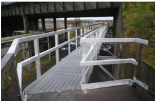
Wilton Steel Works – new Tata Steel Bridge on Teesdale Way in Redcar and Cleveland Borough
